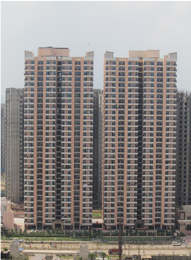
Prasu Infrastructure Pvt. Ltd. S.K.A Green Arch., Greater Noida (West)
