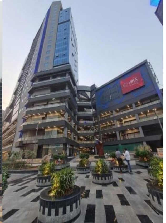
GLD Infra. Project Pvt. Ltd., Galaxy Blue Sapphire Plaza, Greater Noida (West)
